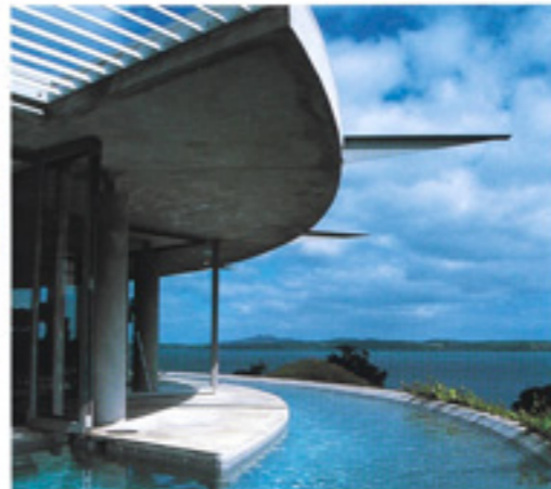
WAIATUA HOUSE, WAIHEKE ISLAND GARNACHAR ARCHITECTS LTD
